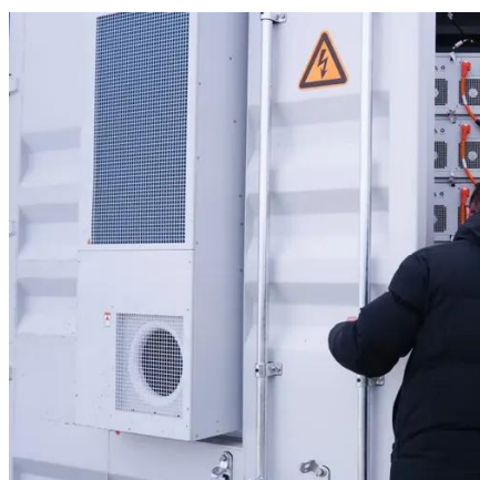
600 800mm Depth Floor Standing Network Server ...
