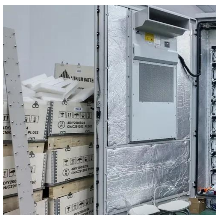
MOBICELL-350 , Hybrid Solar Battery System with 350W Fuel-Cell Cabinet
