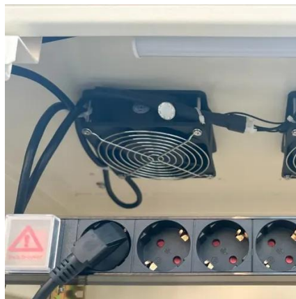
Deye 50kw and 60kw battery bank cabinet #solar energy storage ...
