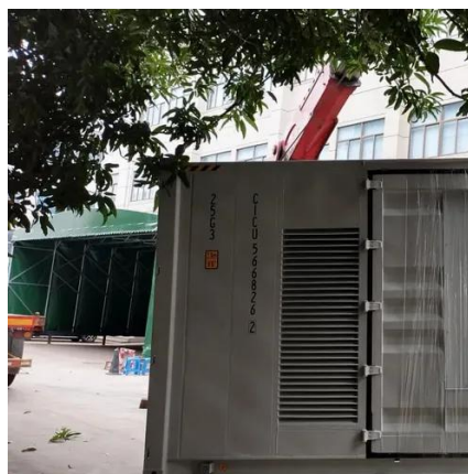
Photovoltaic energy storage cabinet installation in Oman
