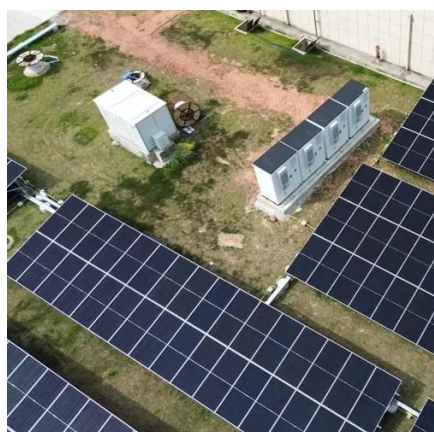
Nickel Cadmium Battery Rack, Battery Rack, NiCd Battery Rack
