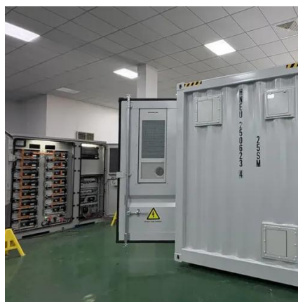
30 kW Solar Kits , SunWatts
