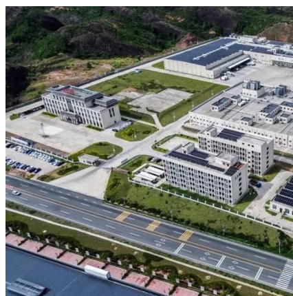
Photovoltaic Grid Cabinet
