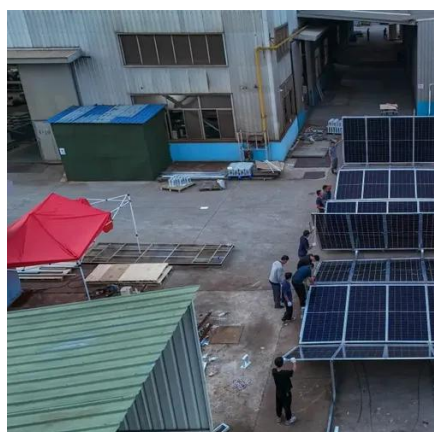
Africa: Demand up for solar coupled with energy storage systems
