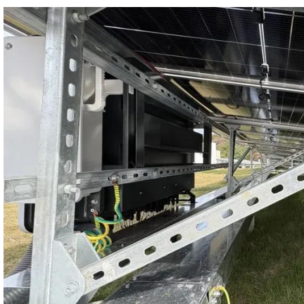
Lithium Ion Energy Storage System 1mwh Hybrid off Grid PV ...
