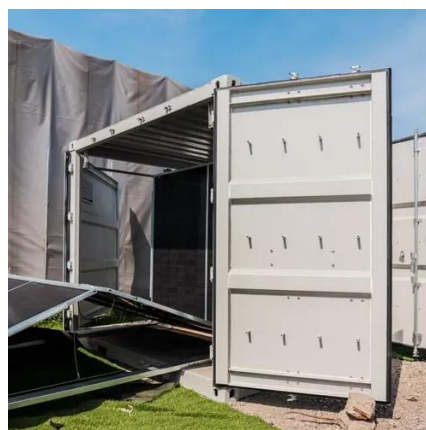
Electric Power Supply Companies in Addis Ababa Ethiopia
